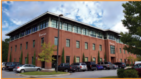
1. North Charleston Medical Pavilion 8992 University Boulevard, North Charleston
